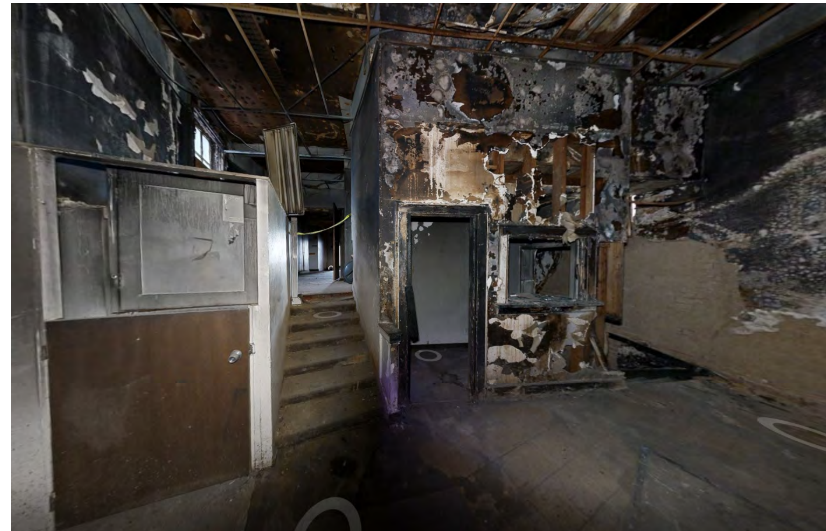
PHOTO_8 WHEELCHAI LIFT
