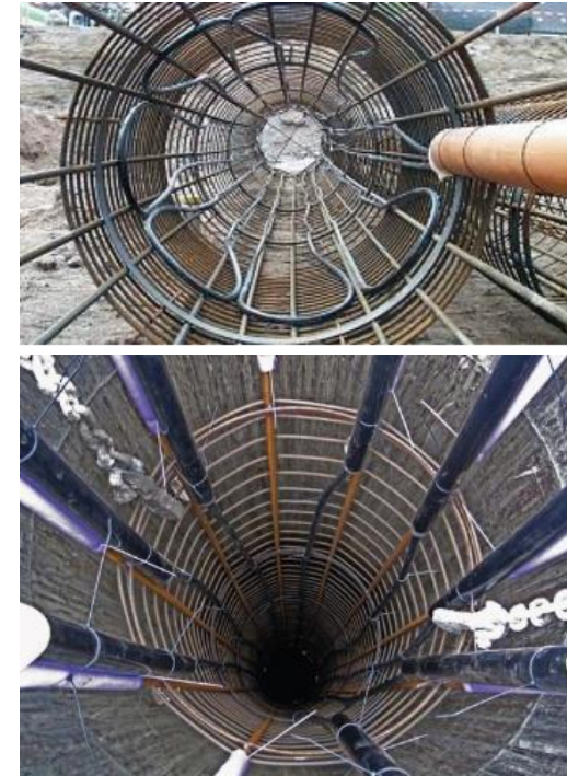
Concrete Pier Example
