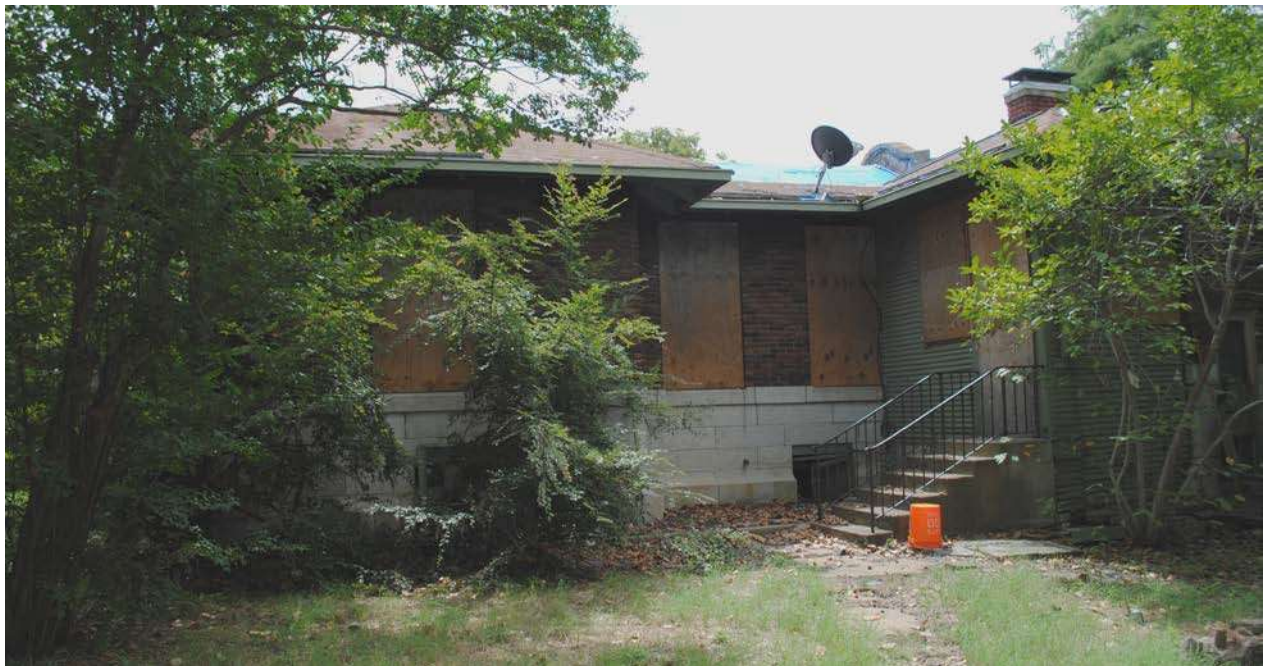
Figure 7. Bianchi House, Northwest Elevation, August 2017
