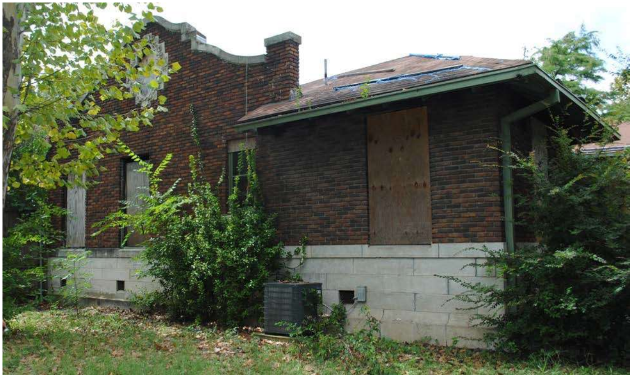
Figure 6. Bianchi House, Northeast Elevation, August 2017
