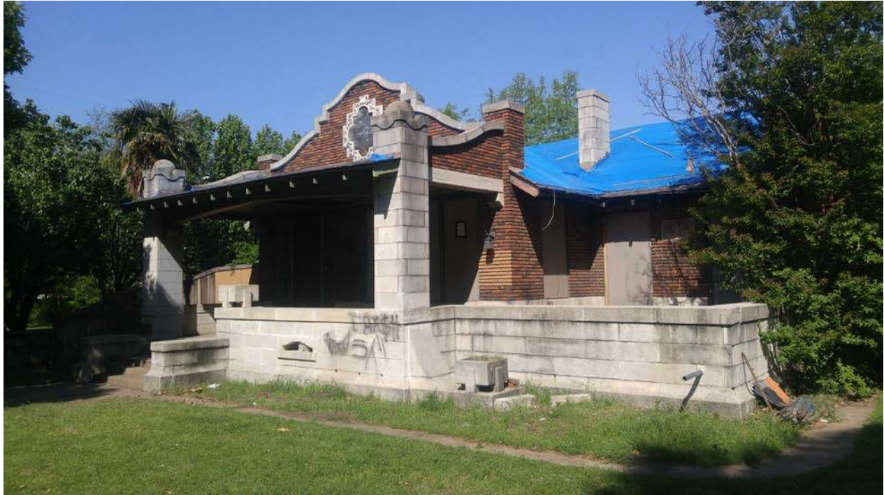
Figure 4. Bianchi House, Southeast Elevation, April 2018
