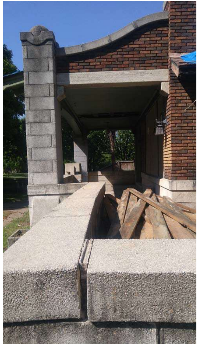
Figure 9. Terrace, looking towards porch
