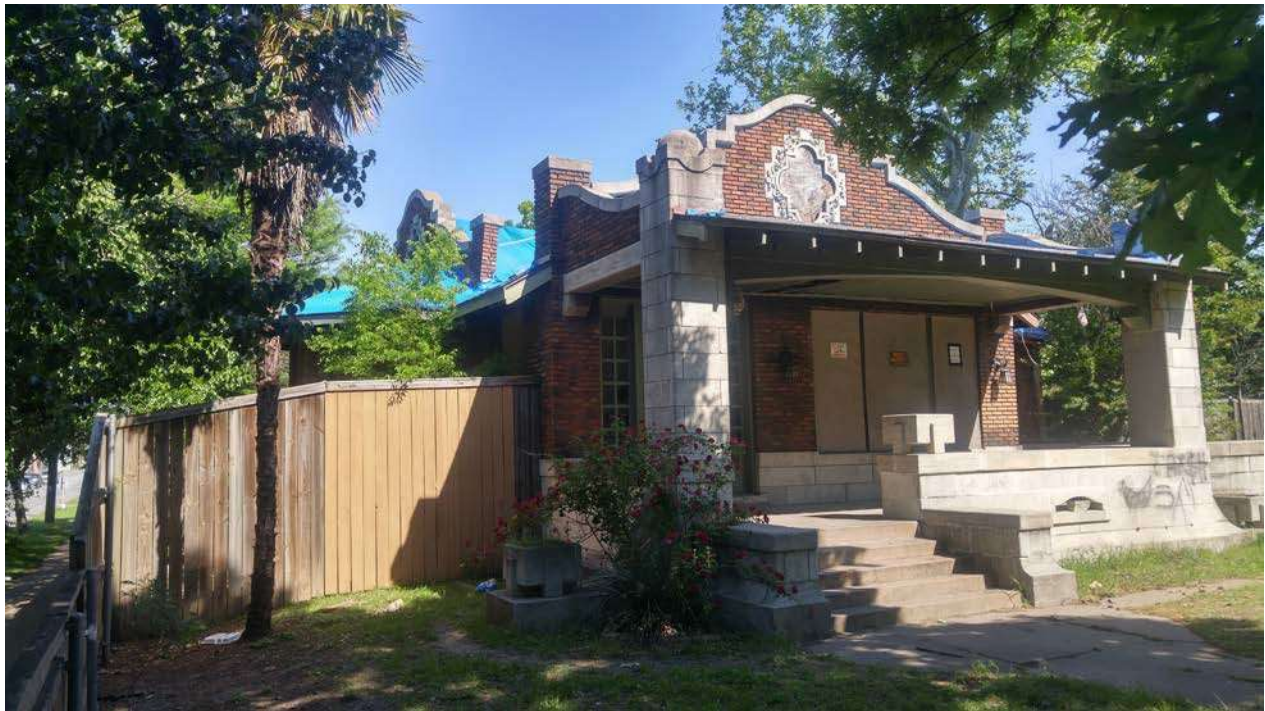
Figure 5. Bianchi House, Southwest & Southeast Elevations, April 2018
