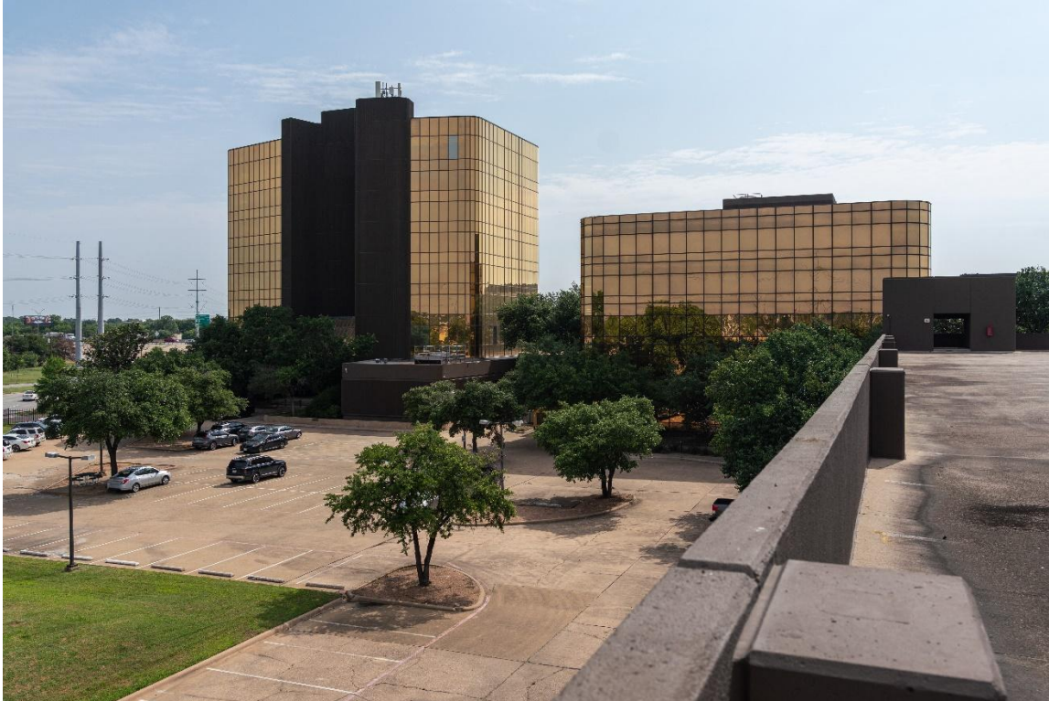
Photo 11: West elevations - Towers 1 & 2 Camera facing east.
