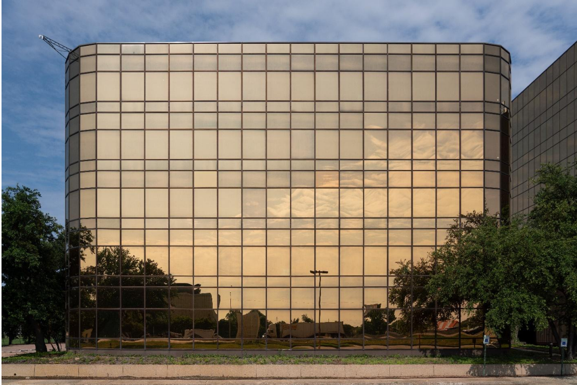
Photo 7: East elevation - Tower 2 Camera facing west.
