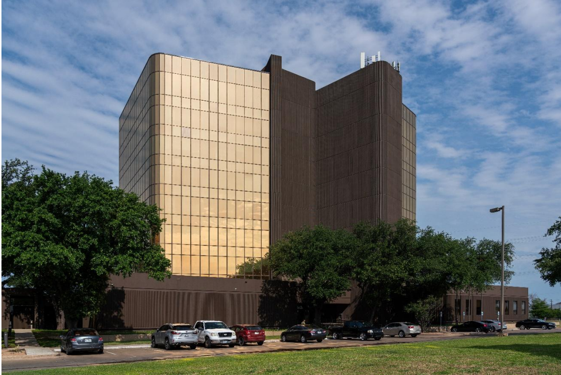
Photo 5: East elevation - Tower 1 Camera facing northwest.
