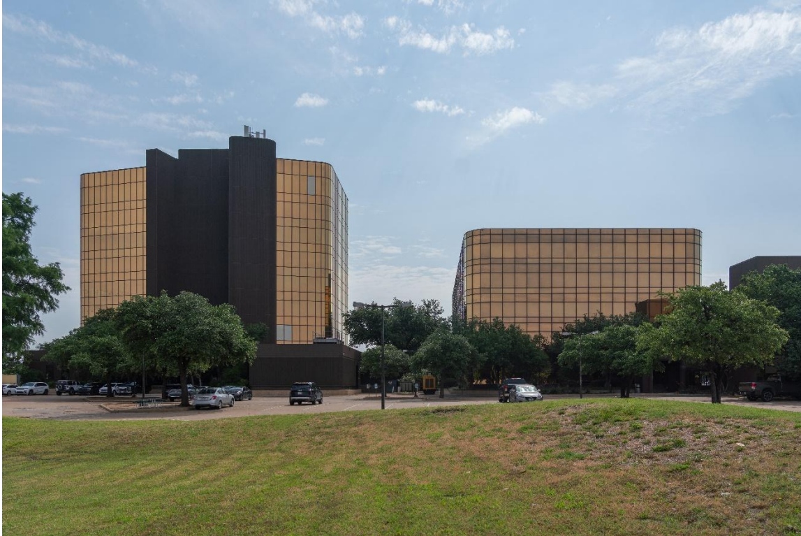
Photo 15: West elevations - Towers 1 & 2 Camera facing east.
