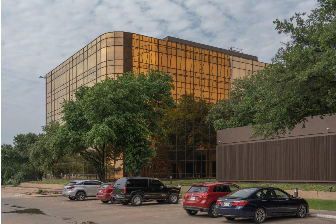
Photo 4: Northeast oblique - Tower 2 Camera facing southwest.
