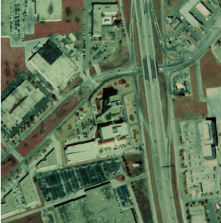
Figure 3: (1989) Mary Kay site 4 years post-construction of Tower 2 and garage. Historic Aerials - Retrieved from Historic Aerials by NETROnline
