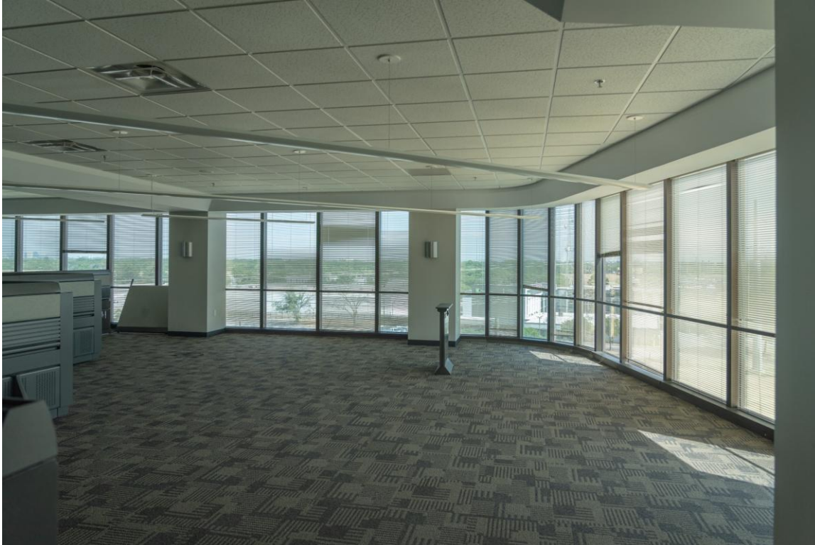
Photo 32: 5 th floor, north side – Tower 1 Camera facing north.
