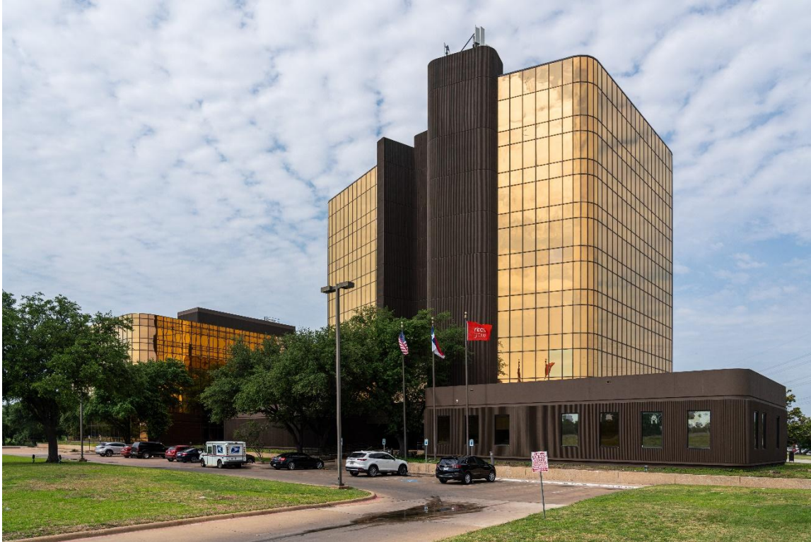
Photo 2: Northeast oblique – Tower 1 Camera facing southwest.
