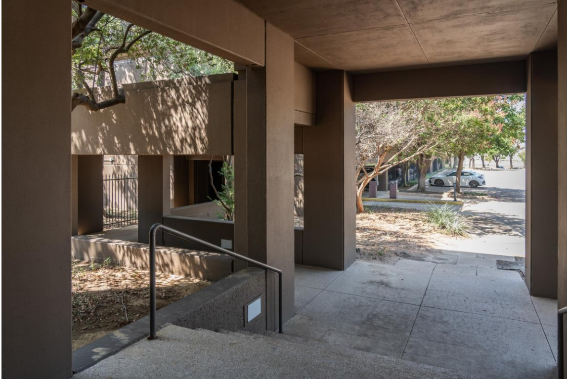
Photo 41: Covered walkway to garage – Tower 2 Camera facing west.
