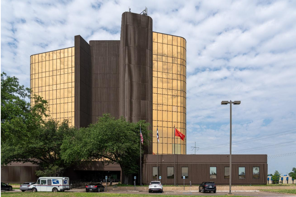
Photo 3: East elevation - Tower 1 Camera facing west.
