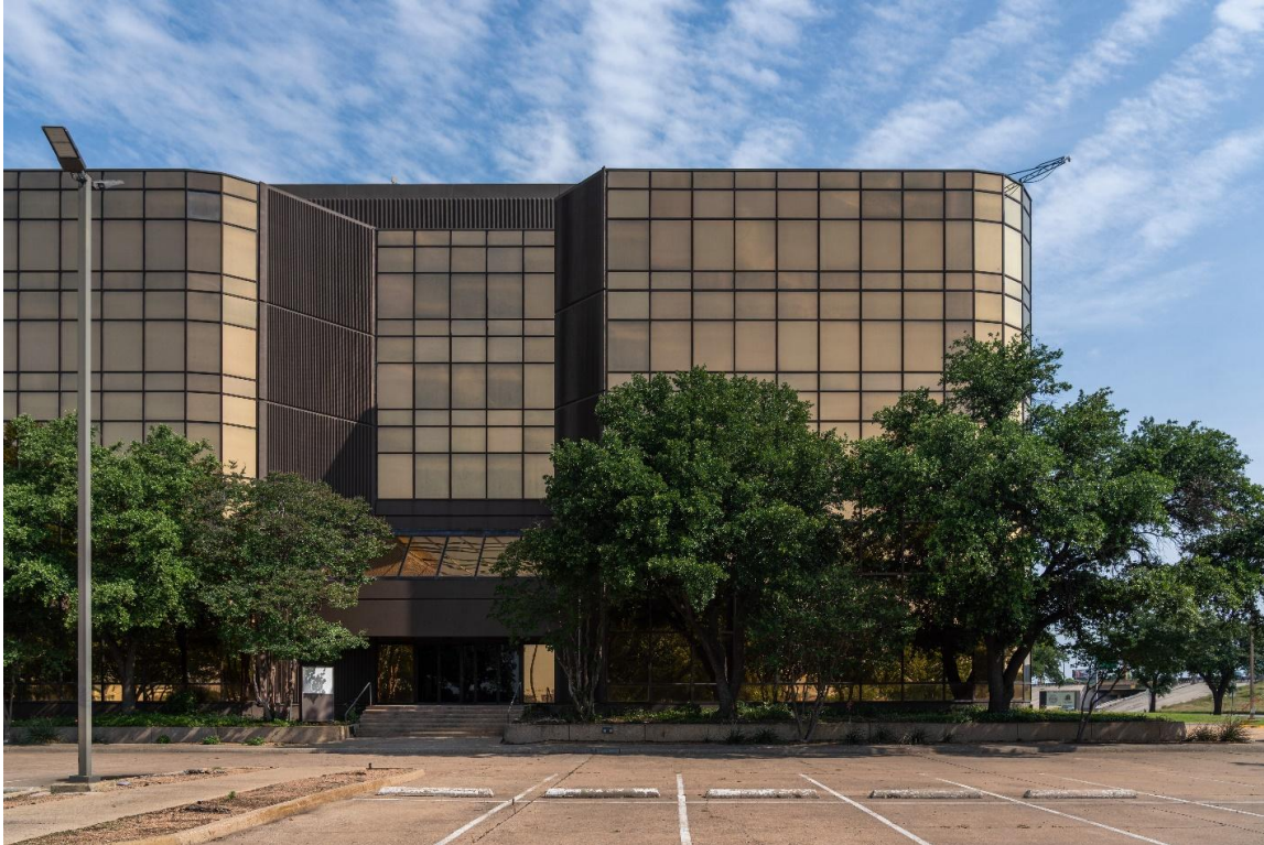
Photo 9: South entrance - Tower 2 Camera facing north.
