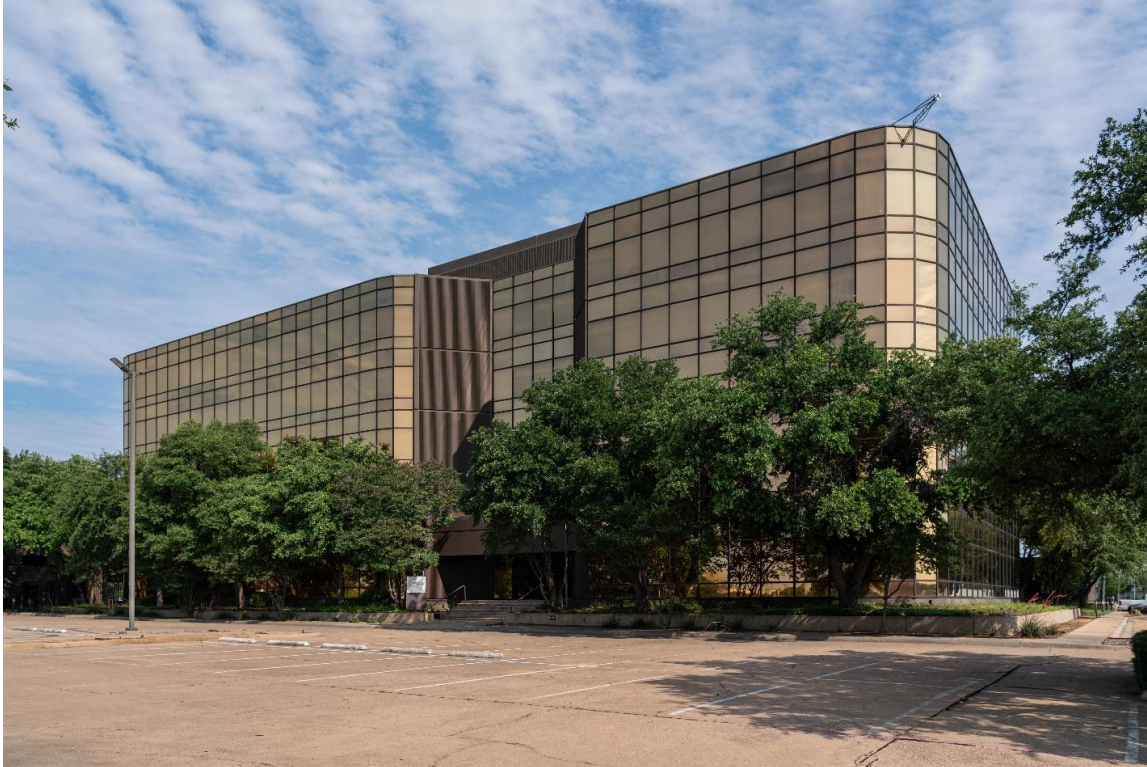
Photo 8: South elevation - Tower 2 Camera facing northwest.
