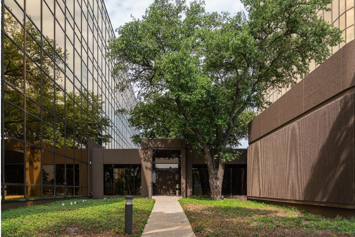
Photo 19: East elevation of breezeway between Tower 1 and Tower 2 Camera facing west.
