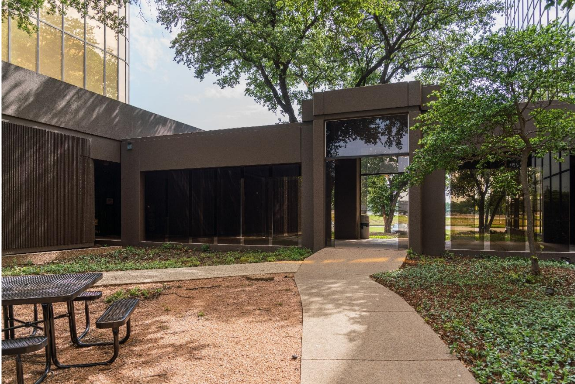
Photo 17: West elevation of connecting breezeway Camera facing east.
