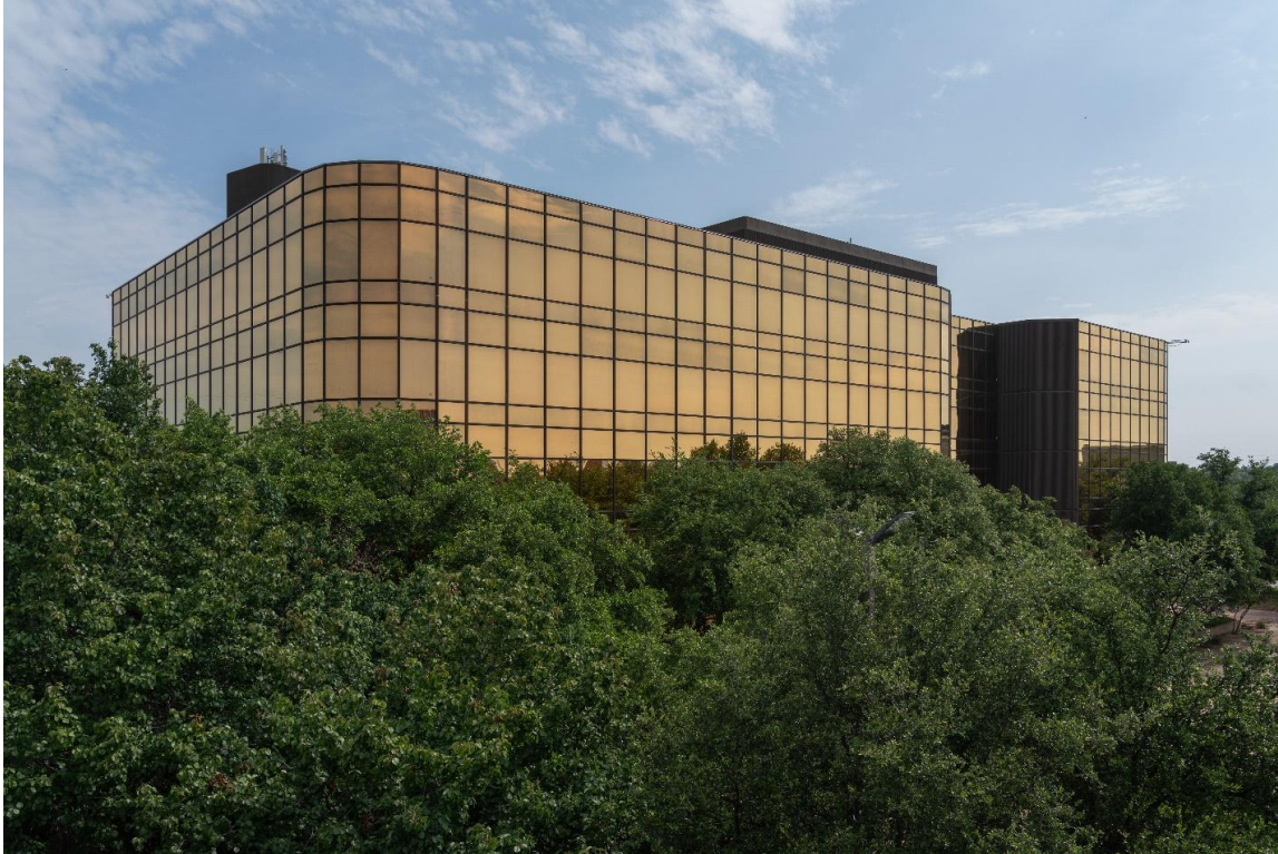
Photo 10: Southwest oblique - Tower 2 Camera facing northeast.
