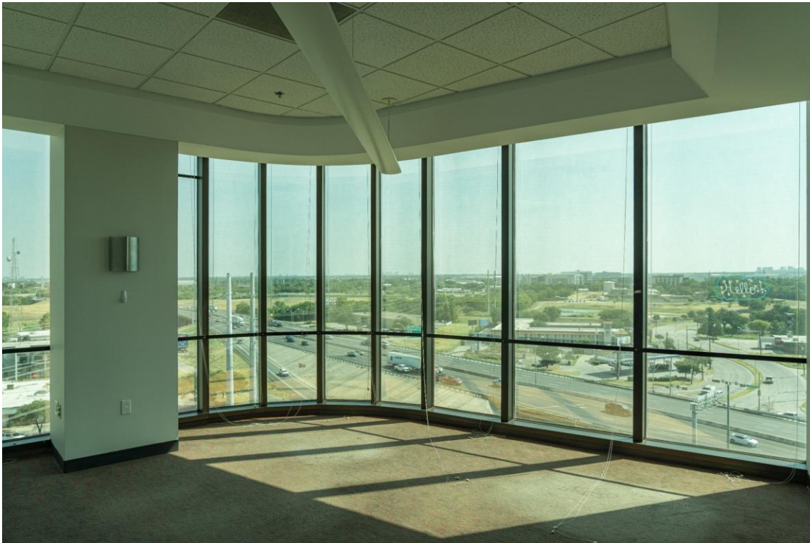
Photo 37: 8 th floor northeast corner office – Tower 1 Camera facing northeast.
