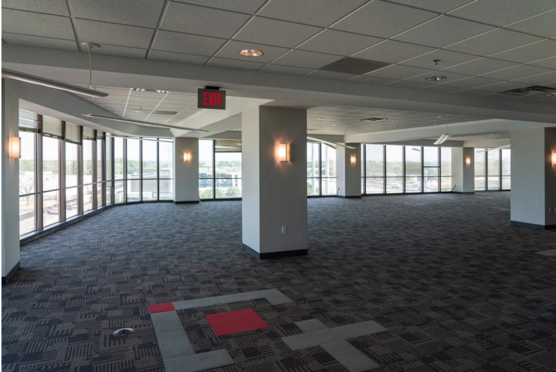
Photo 31: 4 th floor, north side – Tower 1 Camera facing north.
