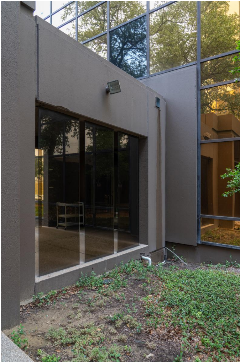
Photo 45: Breezeway at north entrance – Tower 2 Camera facing southeast.
