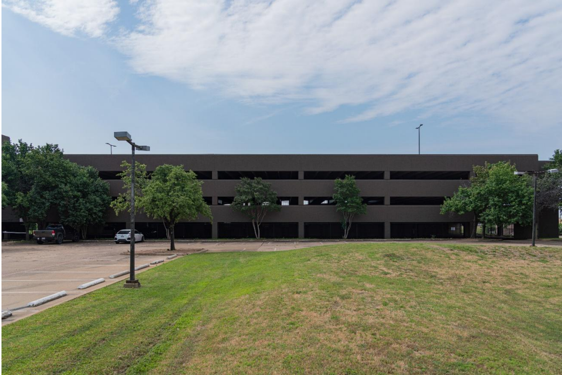
Photo 14: North elevation - Garage Camera facing south.
