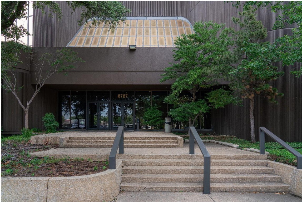
Photo 21: West entrance – Tower 1 Camera facing east.
