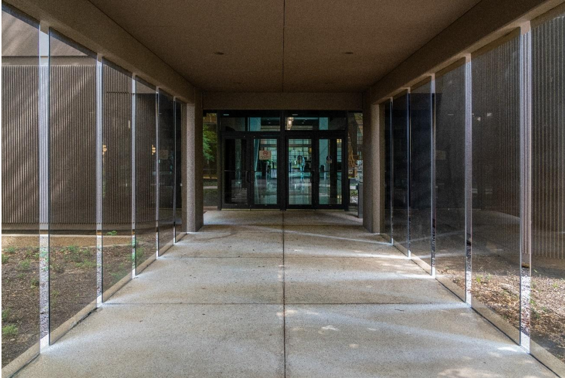
Photo 18: South entrance – Tower 1 Camera facing north.
