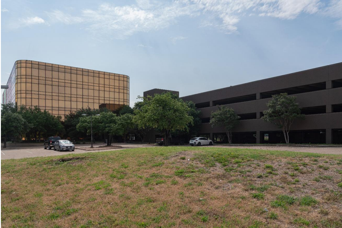
Photo 13: West elevation - Tower 2 & Garage Camera facing east.
