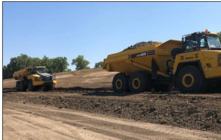
Left: Earth hauling for levee raise; Right; final inspection of west levee prior to O&M turnover
