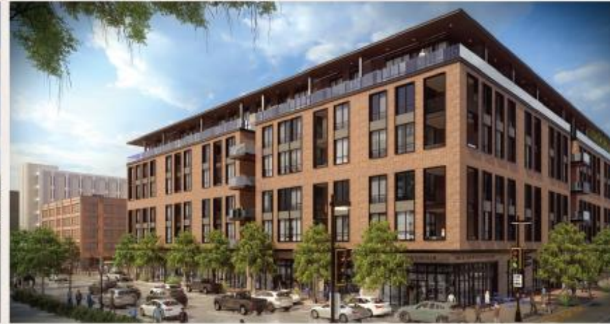
Illustration of new ground-up construction on existing surface lot portion of 805 Elm Street
