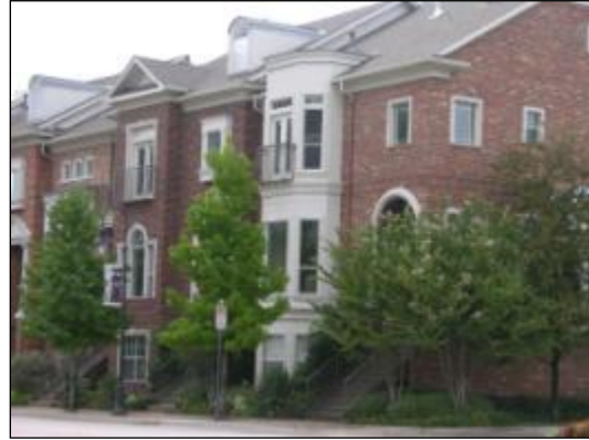
Camden Phase II - 17 Town Homes
