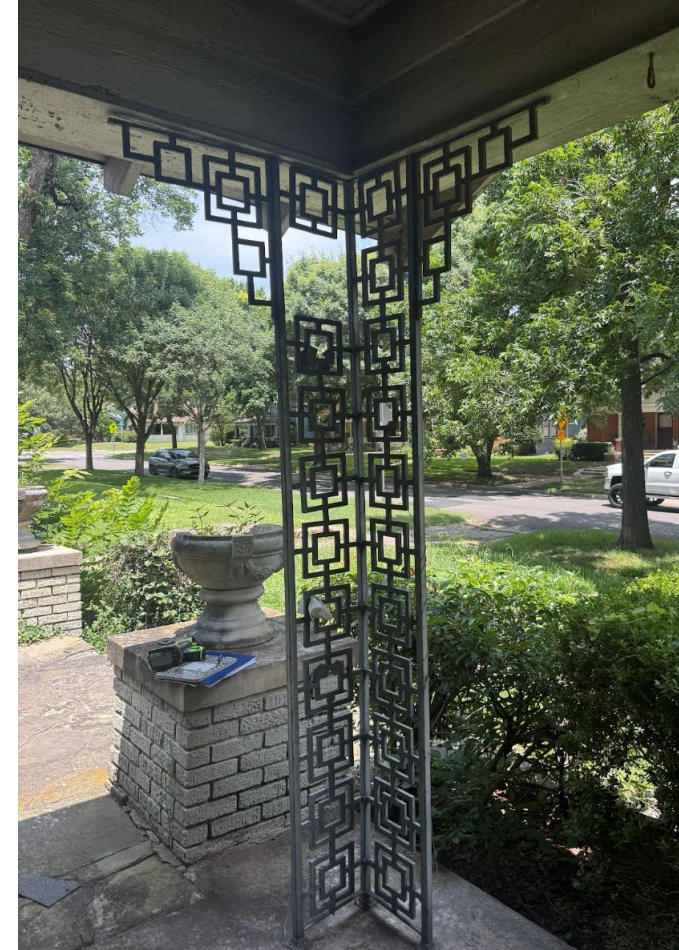
Steel design columns on patio
