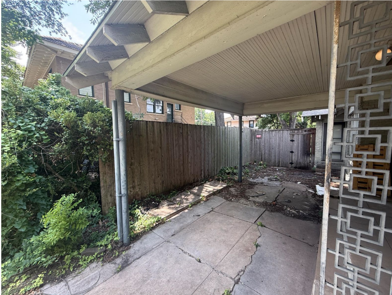
Carport / Porte Cochere round steel column
