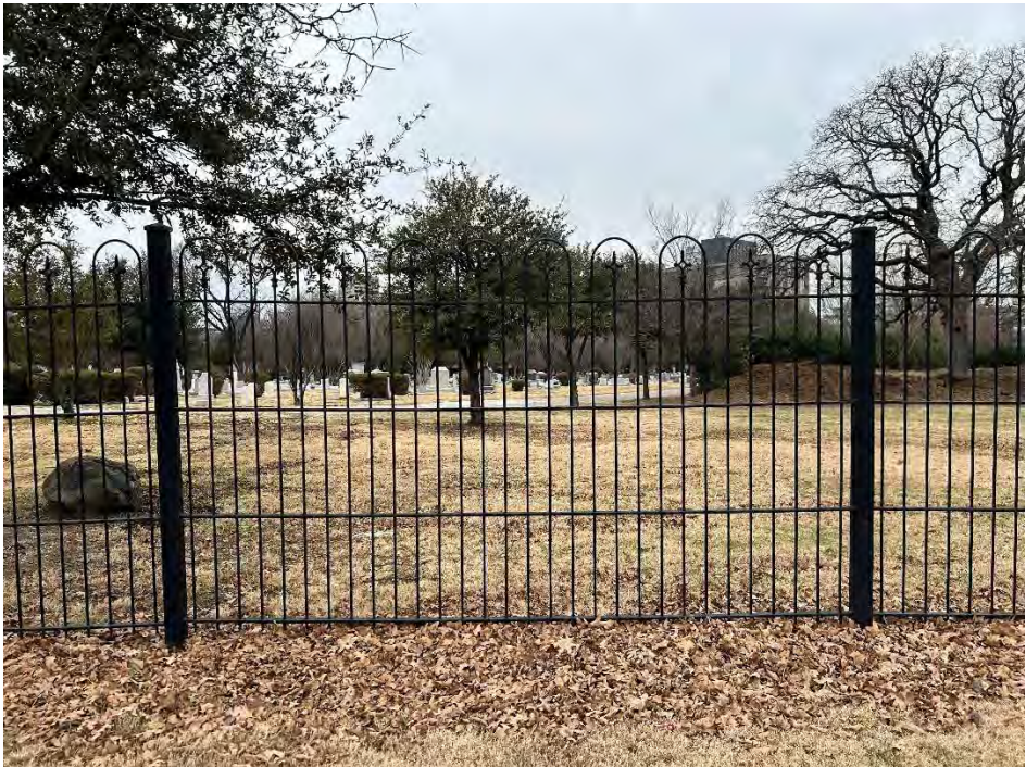
Photograph 8 – Typical existing 6’ tall metal fence that surrounds the Cemetery today: most of this fence will remain in place, and repaired as needed.
