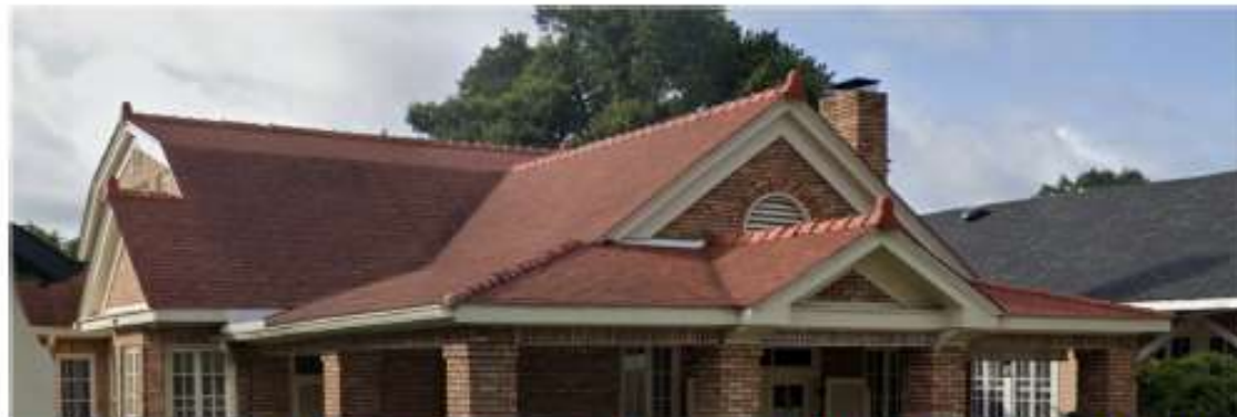
Example: Composition shingles in a color palette of original Spanish tile roofs with terra cotta hips, ridge caps, and rake tiles applied to mimic original tile roofs.
