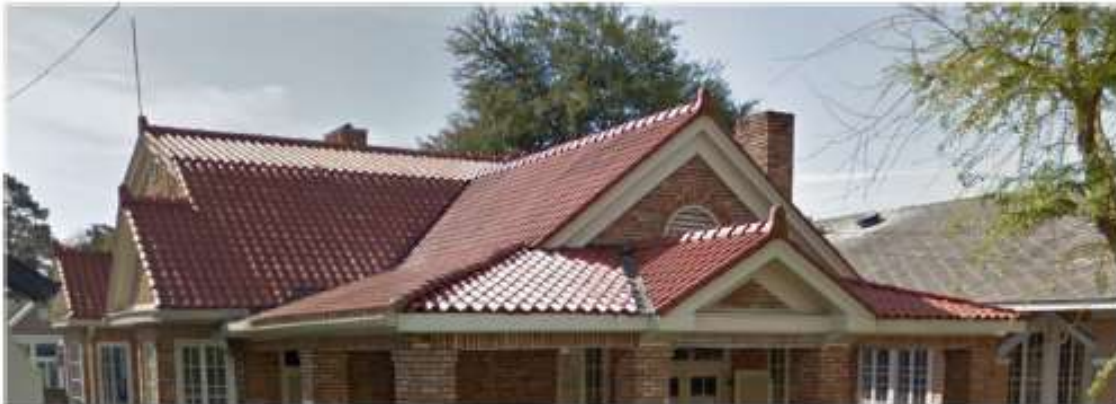
Example: Roof materials that look like Spanish, mission, or barrel style tile in metal, concrete, or plastic composite.
