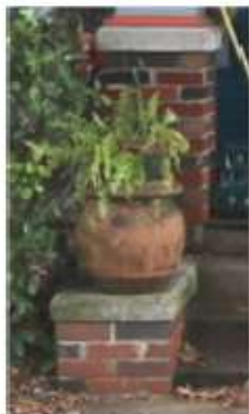
Examples: Square or tapered columns on a brick base with concrete cap.
