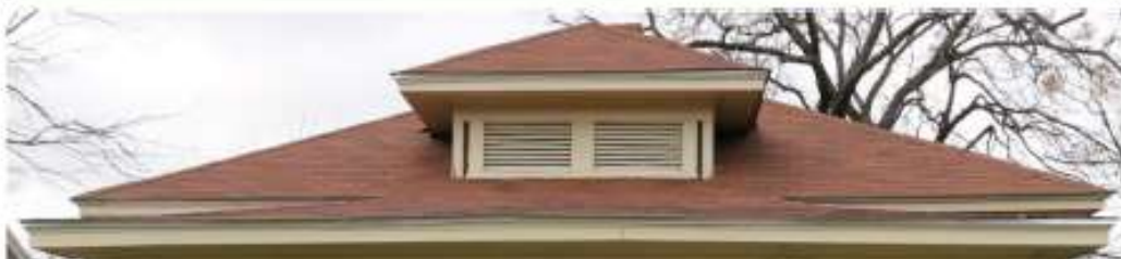
Examples: Centered, hipped dormer with louvered vent.
