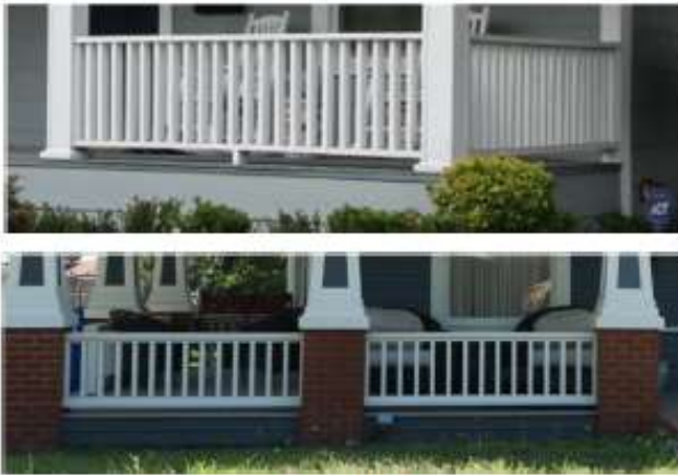
Examples: Wood balustrade on the front porch.
