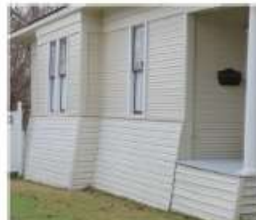
Example: Battered or sloped skirting.
