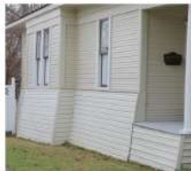
Example: Battered or sloped skirting.
