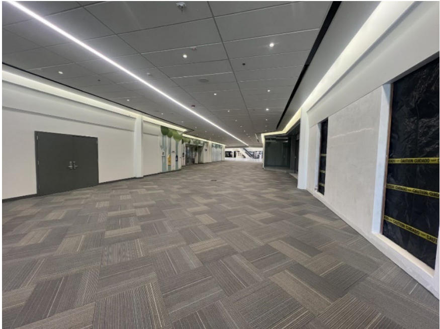
Interior of West Wing improvements - Shops at RedBird
