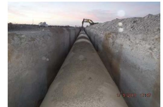
Installation of 108-inch pipe along Section 17
