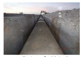
Installation of 108-inch pipe along Section 17
