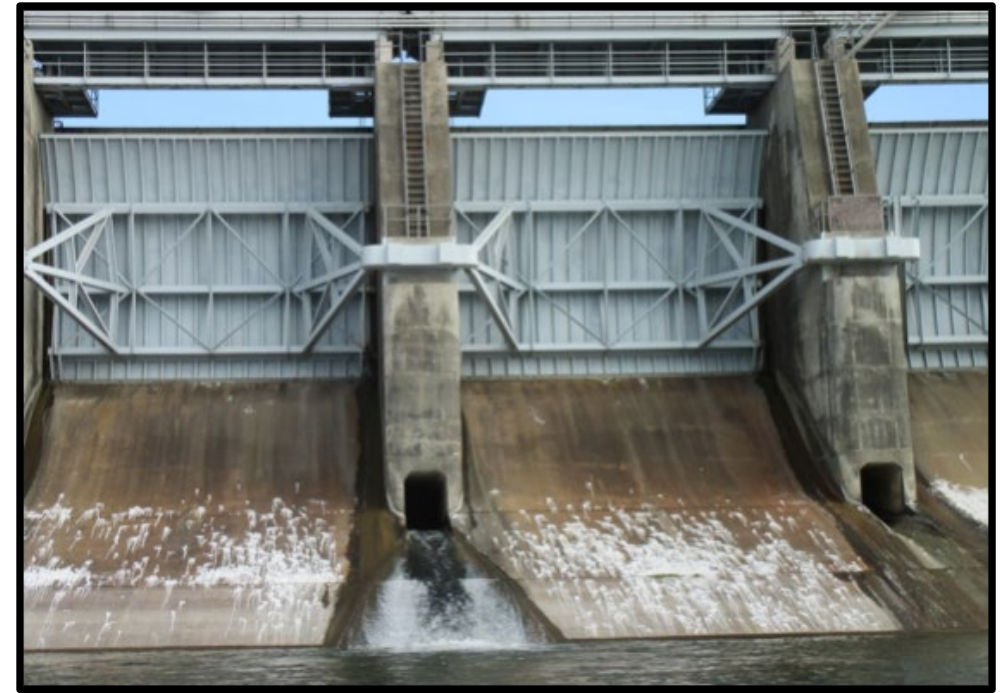
Forney Dam (Lake Ray Hubbard) Tainter Gates
