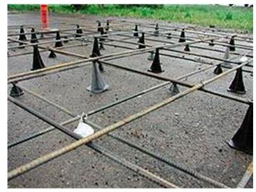
Labor intensive rebar on "chairs" before a concrete pour
