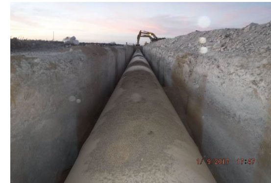
Installation of 108-inch pipe along Section 17
