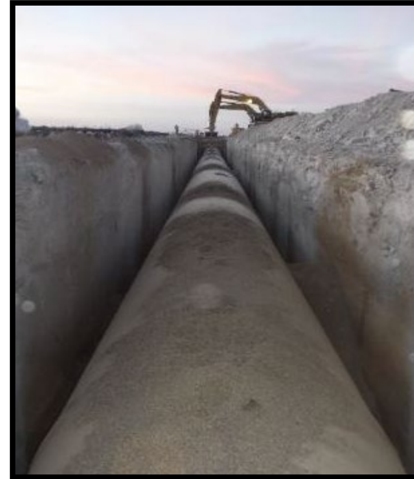
Installation of 108-inch pipe along IPL Section 17
