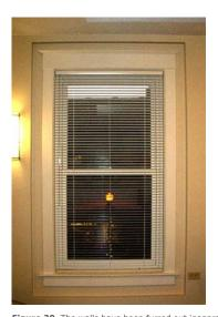
Figure 20. The walls have been furred out inappropriately around the historic window trim creating an appearance the interior never had historically.
