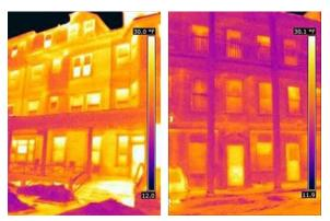
Figure 7.The left thermal image shows the walls of this building before insulating. After insulation was added, the cooler and, thus darker exterior walls evidence how much the heat loss has been reduced. Photos: EYP Architecture & Engineering.
