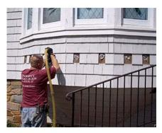
Figure 18. Dense-packed cellulose insulation is being blown in through holes drilled in the sheathing. Once the operation has been completed, the shingles will be reinstalled. Photo: Edward Minch.
