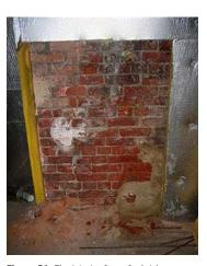
Figure 21. The interior face of a brick masonry wall shows damage that resulted from the installation of a vapor retardant (foil facing) and thermal insulation. Photo: Simpson Gumpertz & Heger.
