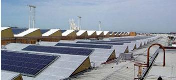
Figure 23. Solar collectors installed in a compatible manner on low sloping sawtooth monitors. Top Photo: Neil Mishalov, Berkeley, CA.
