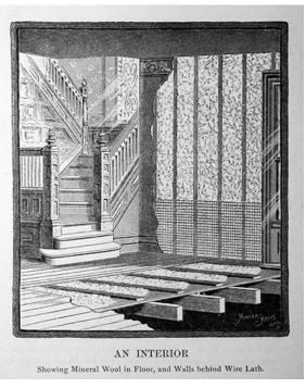
Figure 17. Illustration of insulation from the 1889 trade catalog "The Uses of Mineral Wool in Architecture, Car Building and Steam Engineering". Collection Centre Canadien d'Architecture/Canadian Centre for Architecture, Montreal, Canada.
