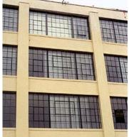
Figure 15. Original steel windows were retained and made operable during the rehabilitation of this historic mill complex. Insulated sliding windows were added on the interior to improve energy efficiency.
