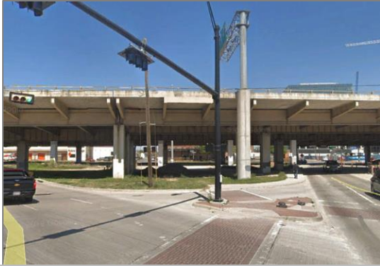
Tunnel portal begins just past Pacific/Cesar Chavez
