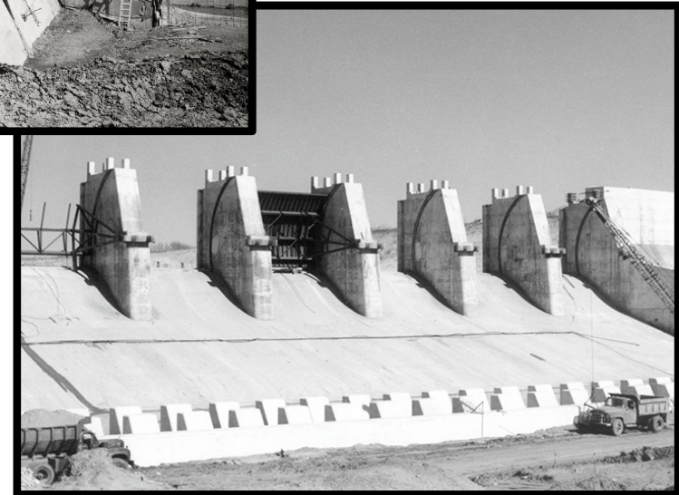
Forney Dam at Lake Ray Hubbard Installation of Tainter Gates
