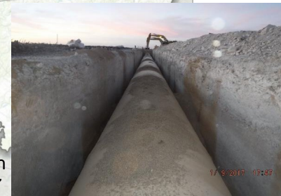
Installation of 108-inch pipe along Section 17
