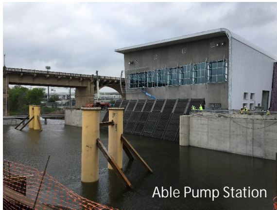
Storm Drainage Debris Removal
