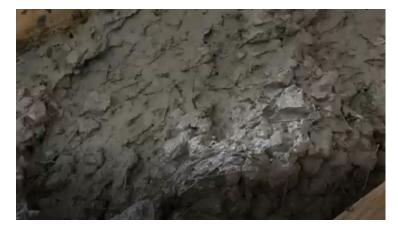
Concrete with fiber mixture ready to be placed with out rebar
