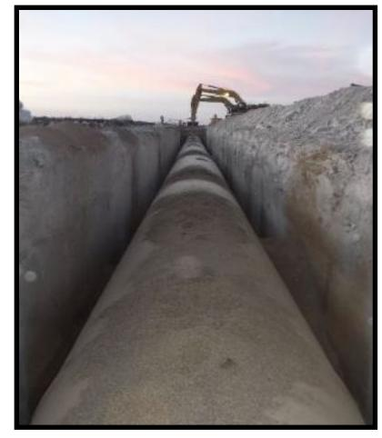
Installation of 108-inch pipe along IPL Section 17
