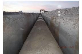
Installation of 108-inch pipe along Section 17
