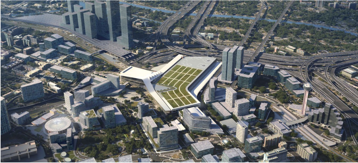
Convention Center Aerial View
