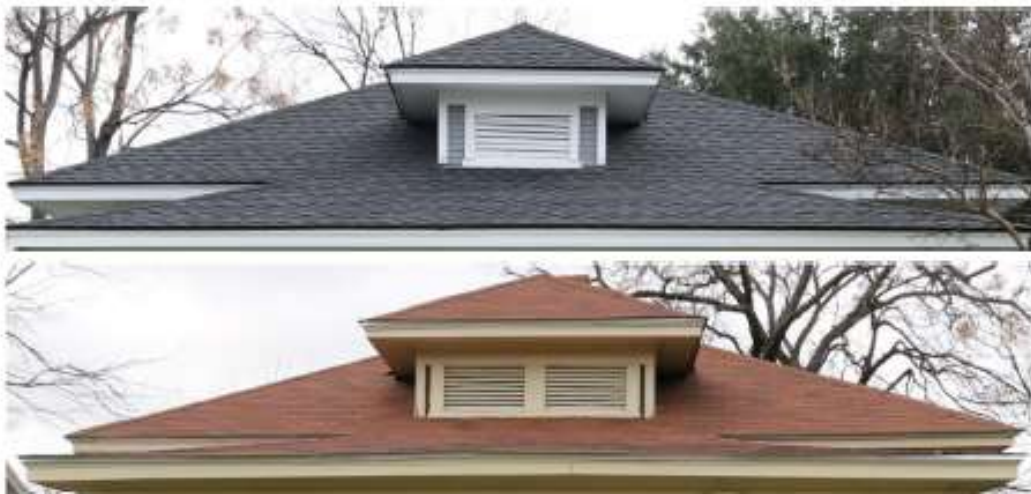
Examples: Centered, hipped dormer with louvered vent.
