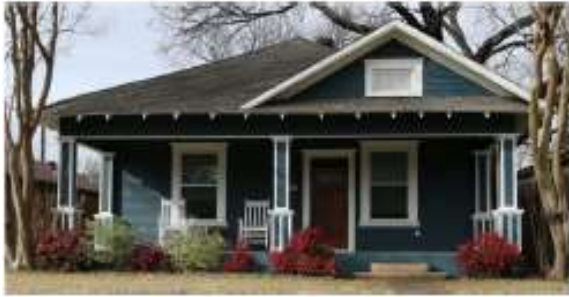
Examples: Recessed gable above the front porch.
