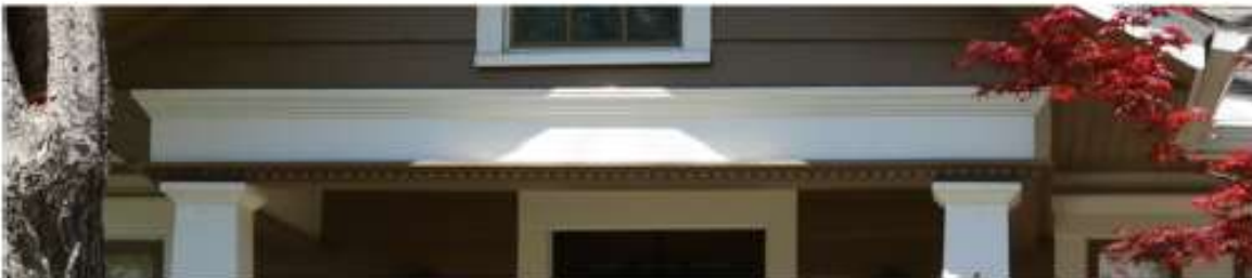
Examples: Minimum 8-inch header beam.
