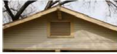
Example: Window or louvered vent centered in front gable.
