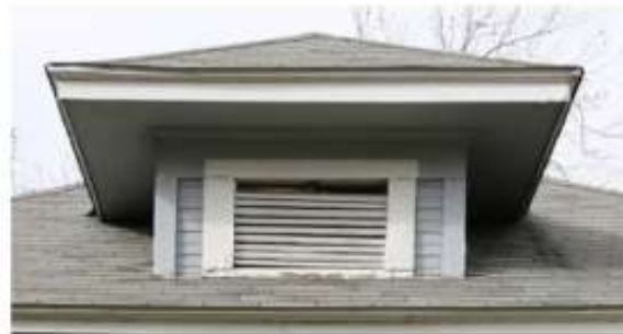
Example: Hipped dormer with louvred vent.
