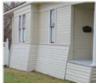
Example: Battered or sloped skirting.
