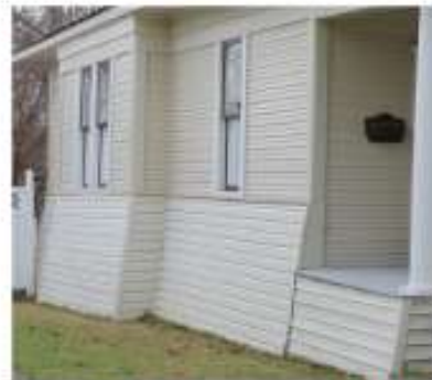
Example: Battered or sloped skirting.
