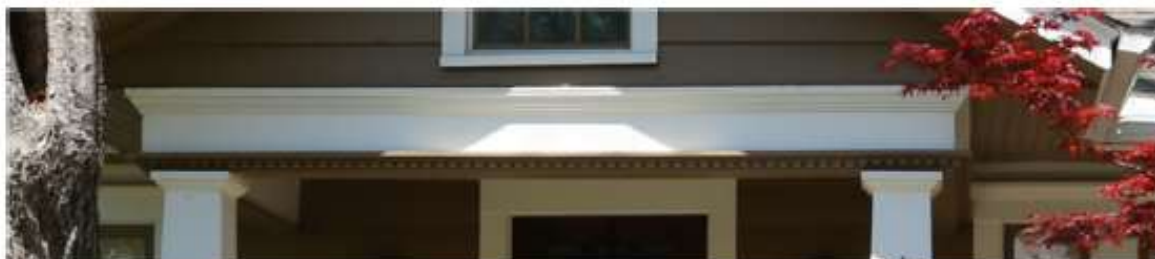
Examples: Minimum 8-inch header beam.
