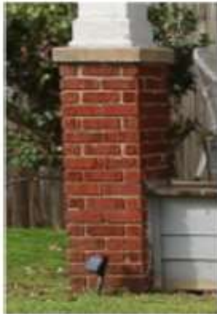
Examples: Square or tapered columns on a brick base with concrete cap.
