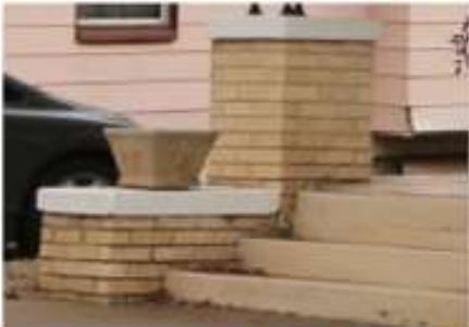
Examples: Wing walls (or cheek wall) on front porch steps.
