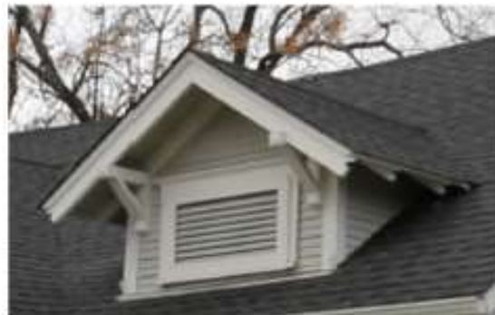
Example: Gabled dormer with louvred vent window.
