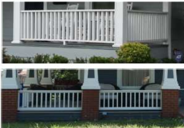
Examples: Wood balustrade on the front porch.
