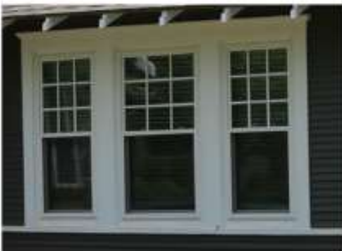
Example: Windows with divided light upper sash.
