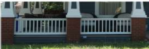
Examples: Wood balustrade on the front porch.
