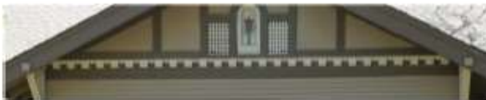
Examples: Dentil molding.
