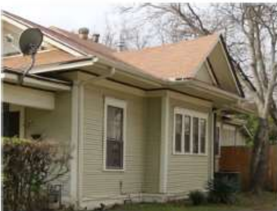
Examples: Projecting bay on side elevation.
