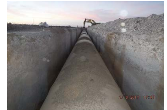
Installation of 108-inch pipe along Section 17
