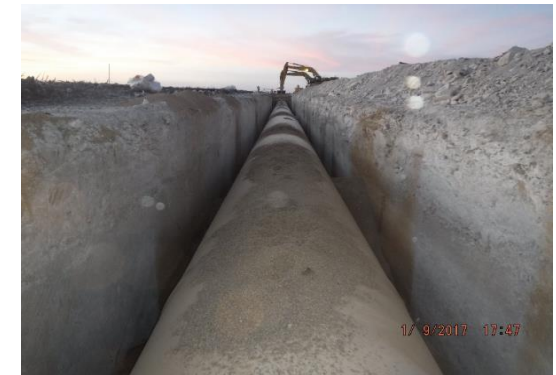
Installation of 108-inch pipe along Section 17
