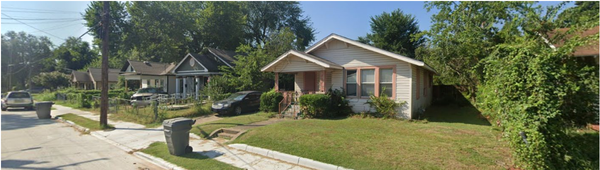
Left (southeast) of subject property on the same blockface. Source: Google Maps -- Streetview.
