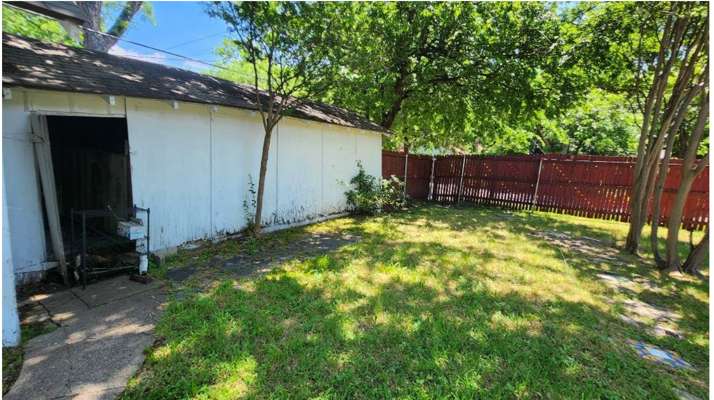
Backyard Interior West Side – Storage Area access. Between Garage/Framed Shed (On Slab) and Framed Shed (No Slab)
