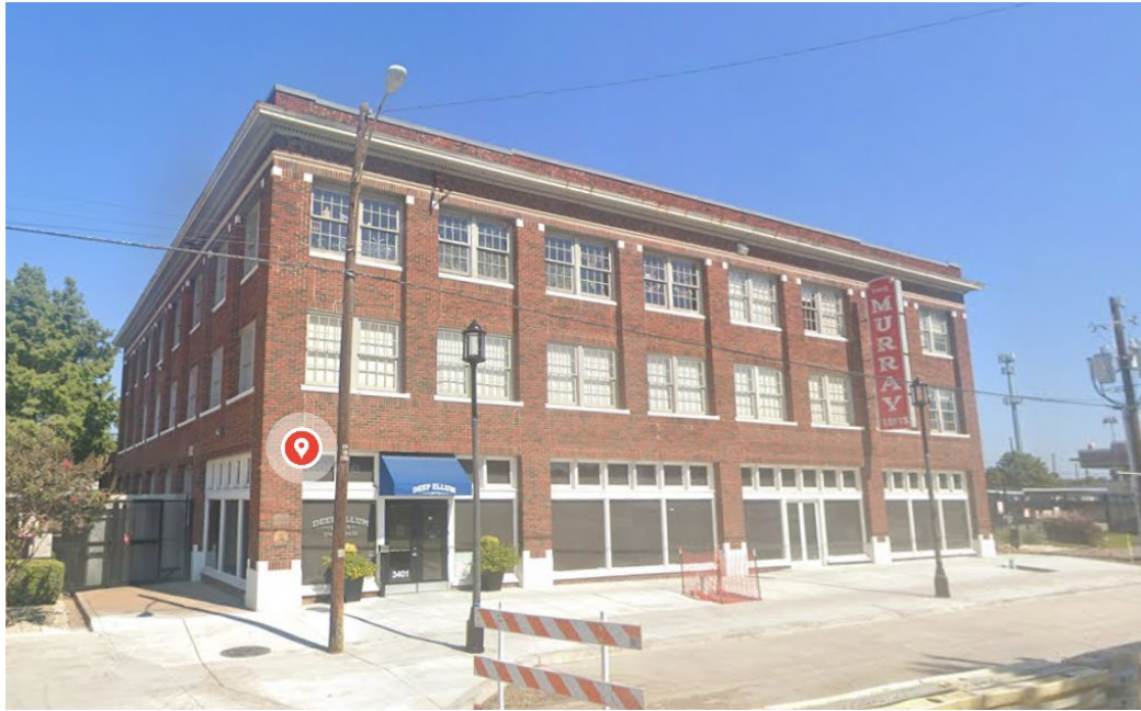
Subject Property: Front façade (south) – main entrance on Commerce St. Source: Google Maps -- Streetview.
