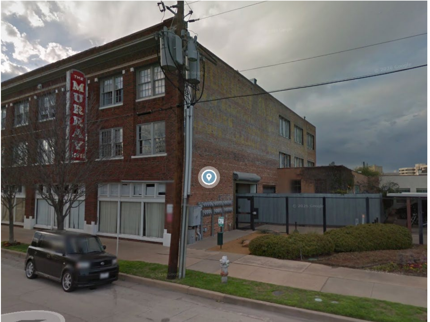
Subject Property: Left (east) elevation. Source: Google Maps -- Streetview.
