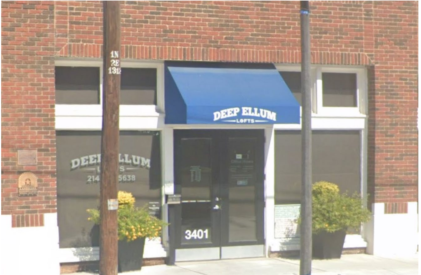
Subject Property: Close up of existing west entrance (wood) double doors. Source: Google Maps -- Streetview.
