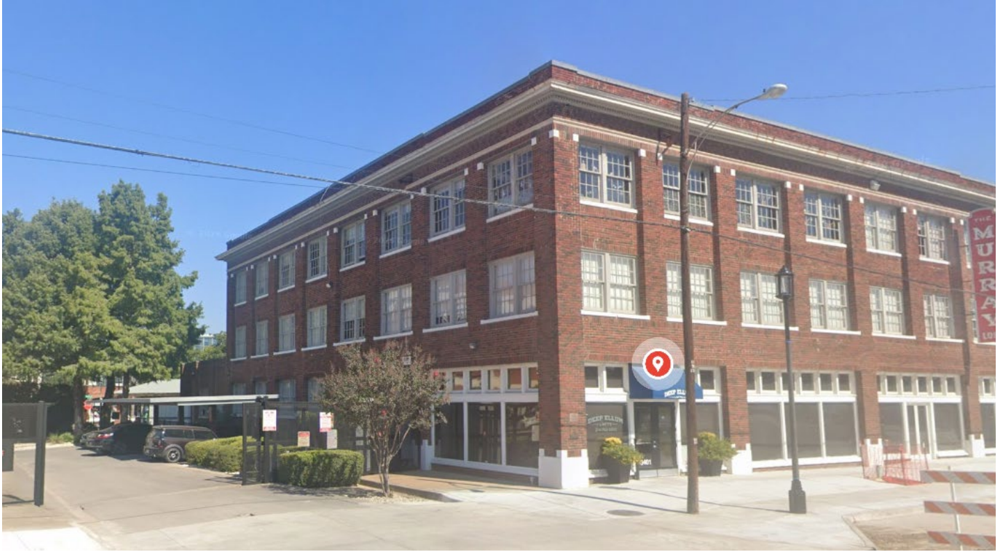
Subject Property: Left (west) elevation. Source: Google Maps -- Streetview.
