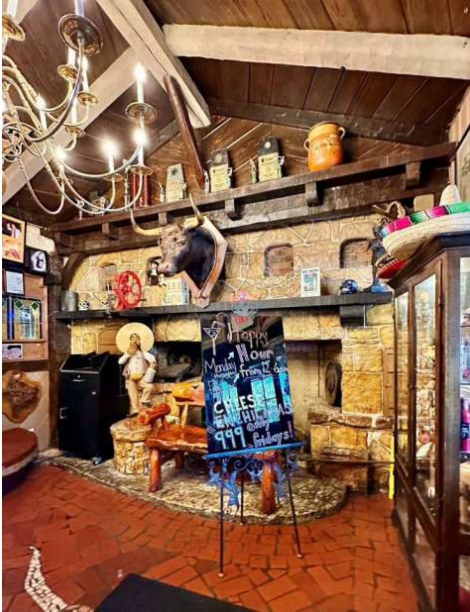
Figure 8. Original barbeque pit, wall and ceiling finishes. Photo courtesy of Willis Winters, FAIA.
