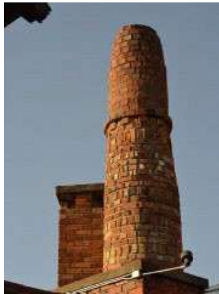
Figure 2. Detail of Chimney. Courtesy of David Preziosi.
