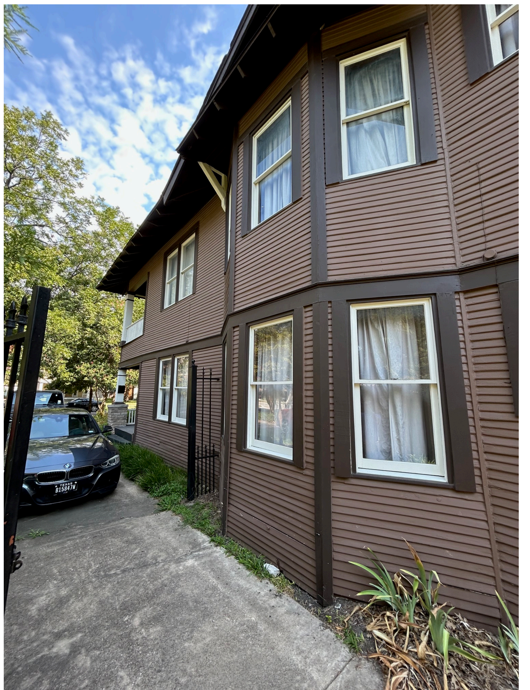
Right (NE) side of main structure
