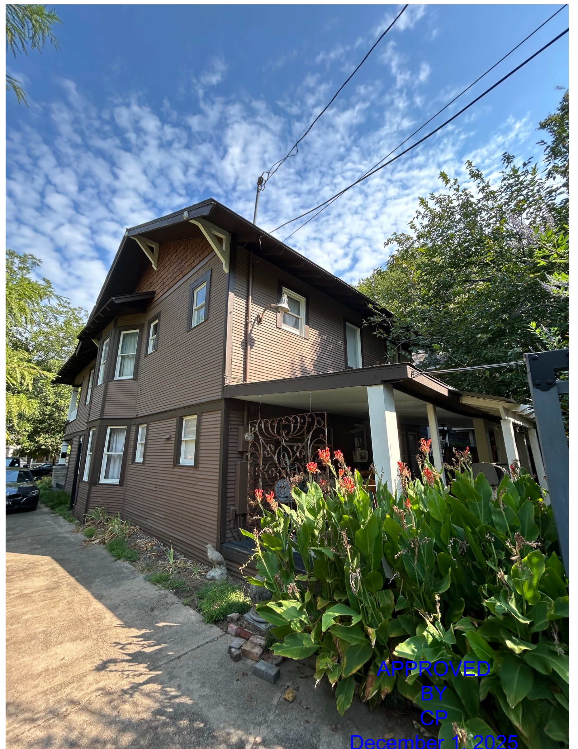
Right (NE) side of main structure from rear
