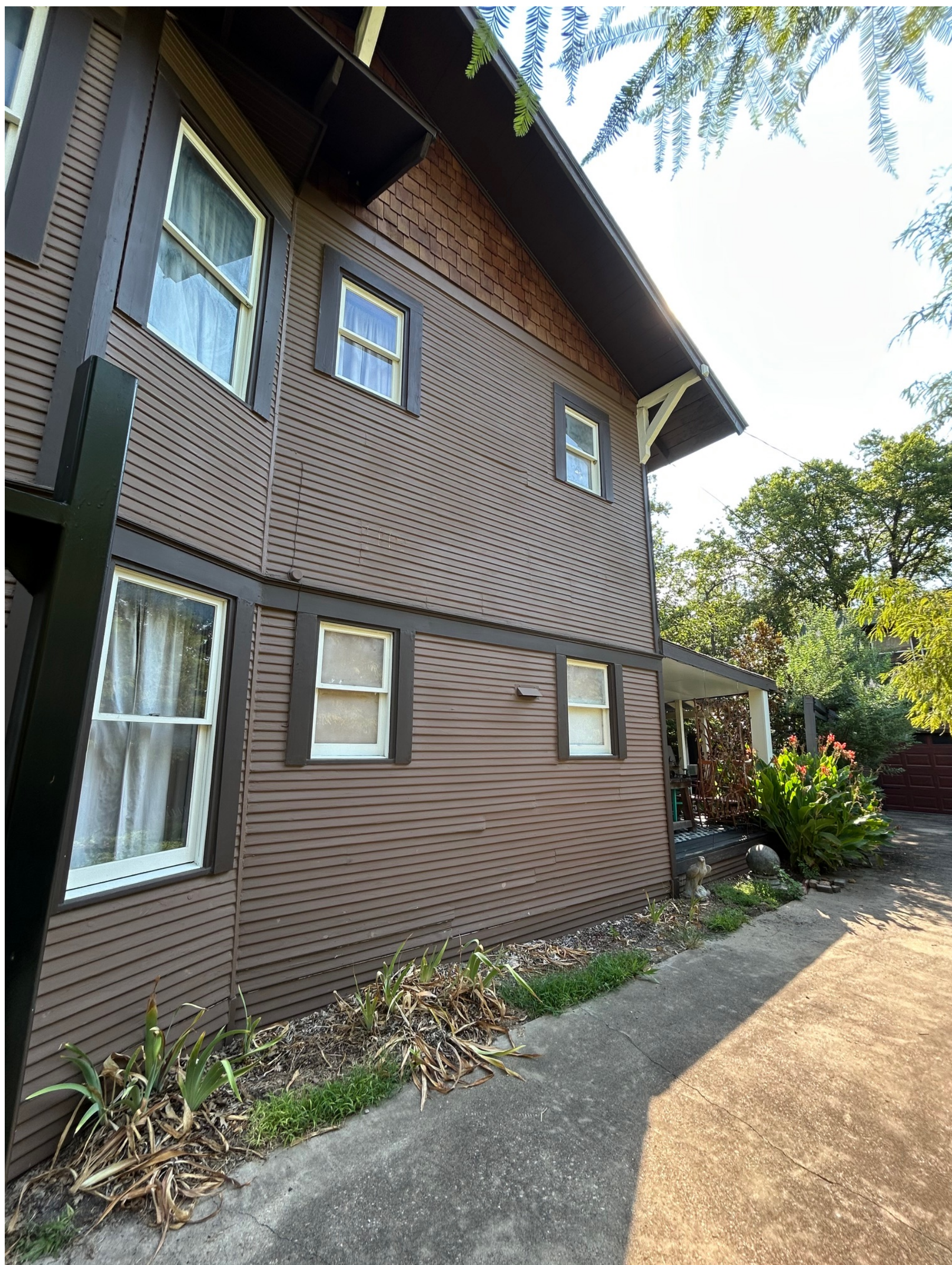
Right (NE) side of main structure
