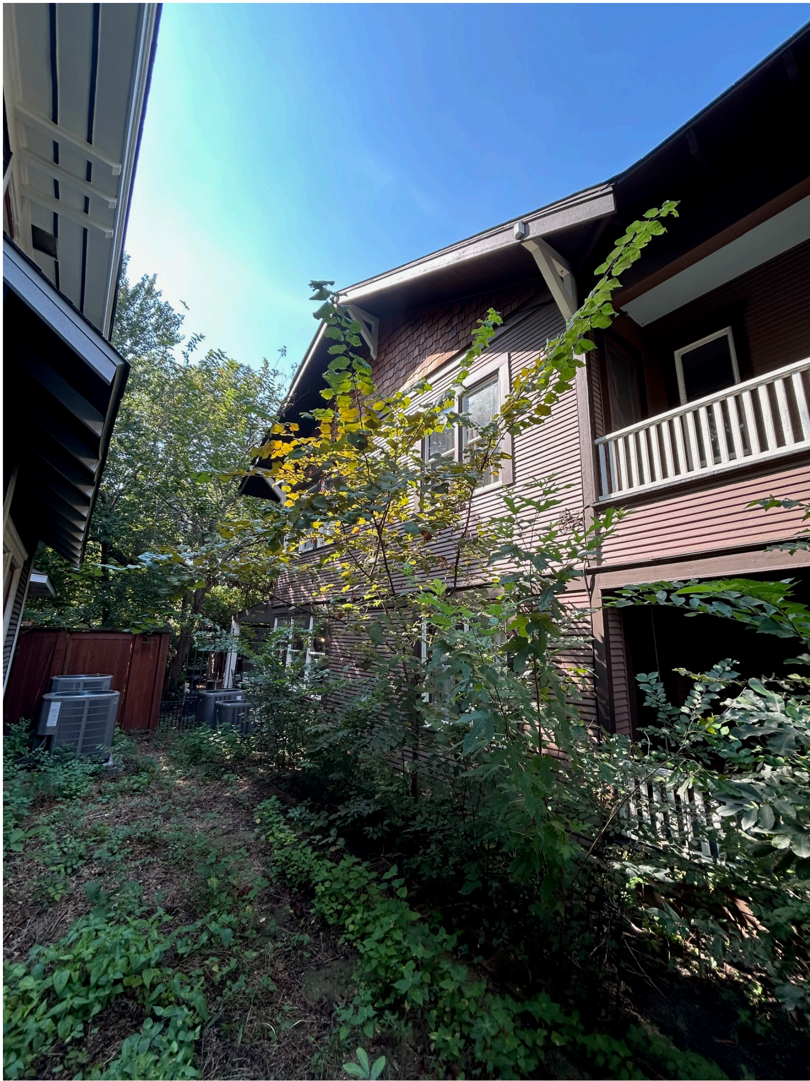
Right (SW) side of main structure
