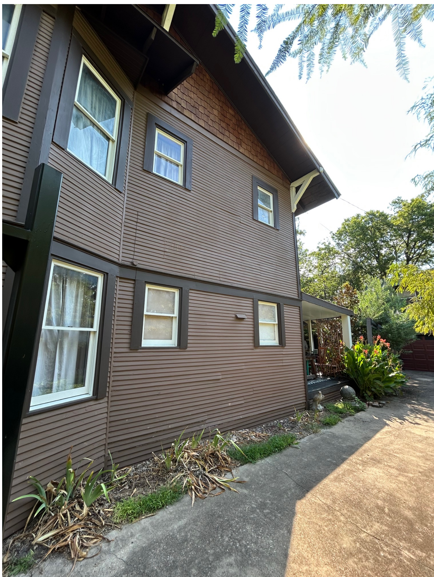
Right (NE) side of main structure
