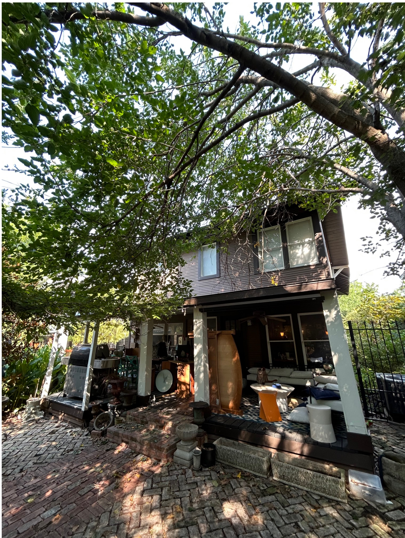
Rear (NW) side of main structure
