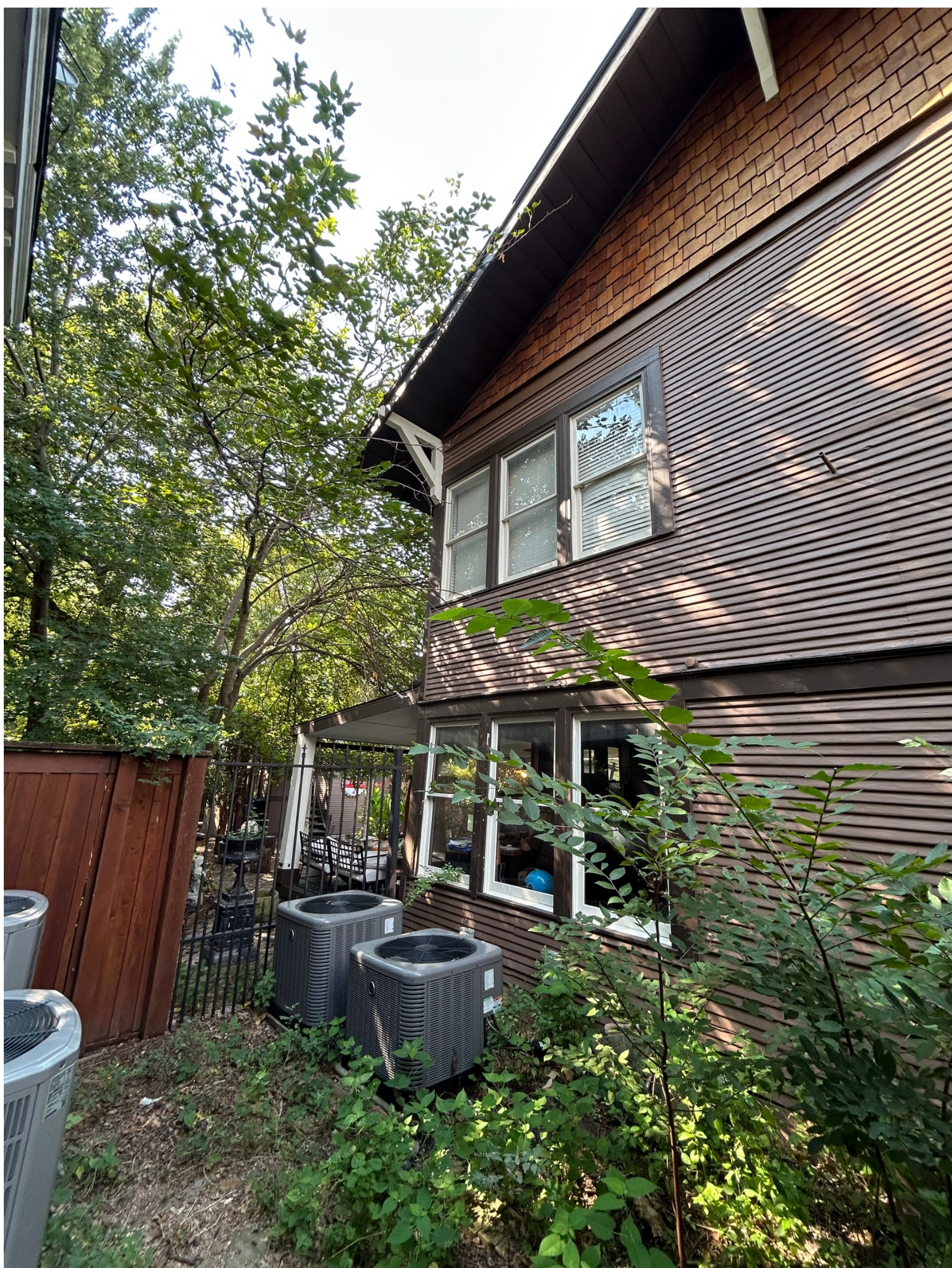
Right (SW) side of main structure
