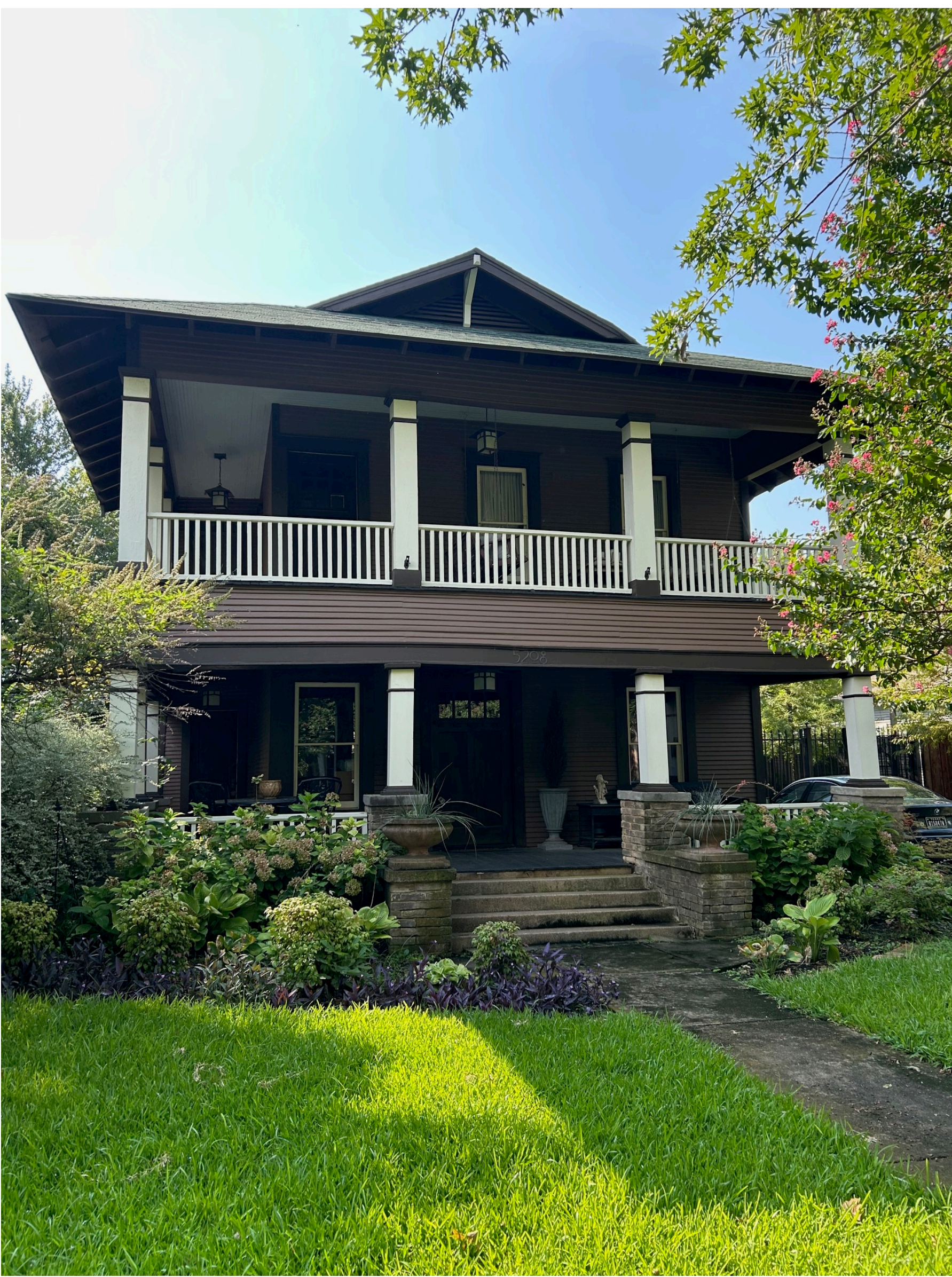
5208 Worth Street - Front Facade
