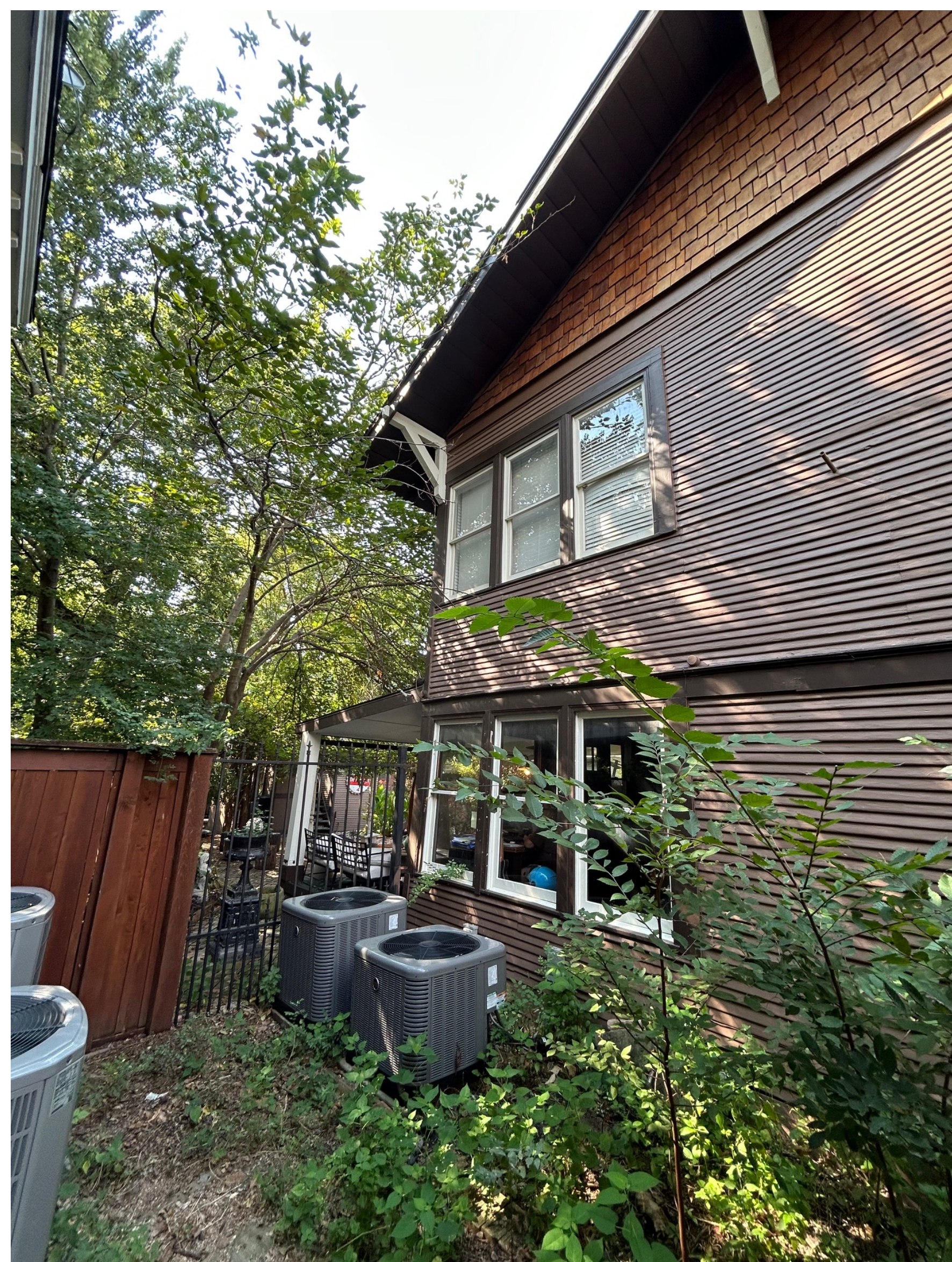
Right (SW) side of main structure
