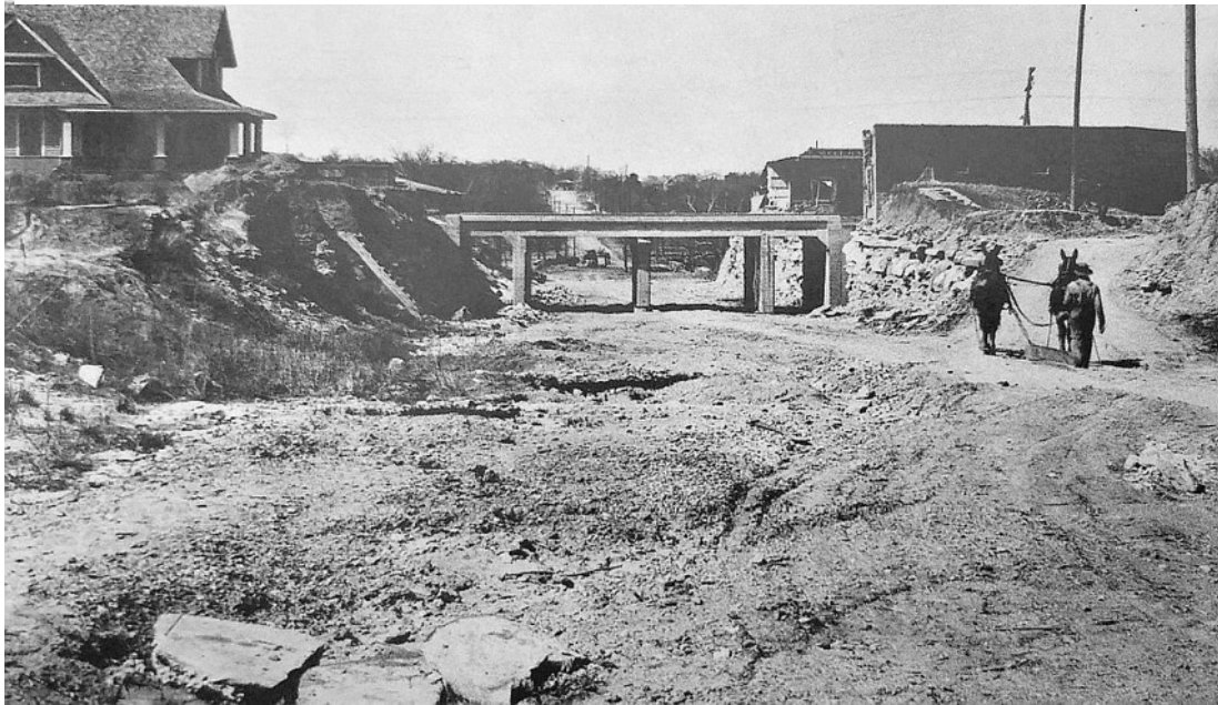
Figure 4- Maple Avenue facing west toward the new Maple/MKT overpass c1918 Dallas Public Library Dallas History and Archives Division
